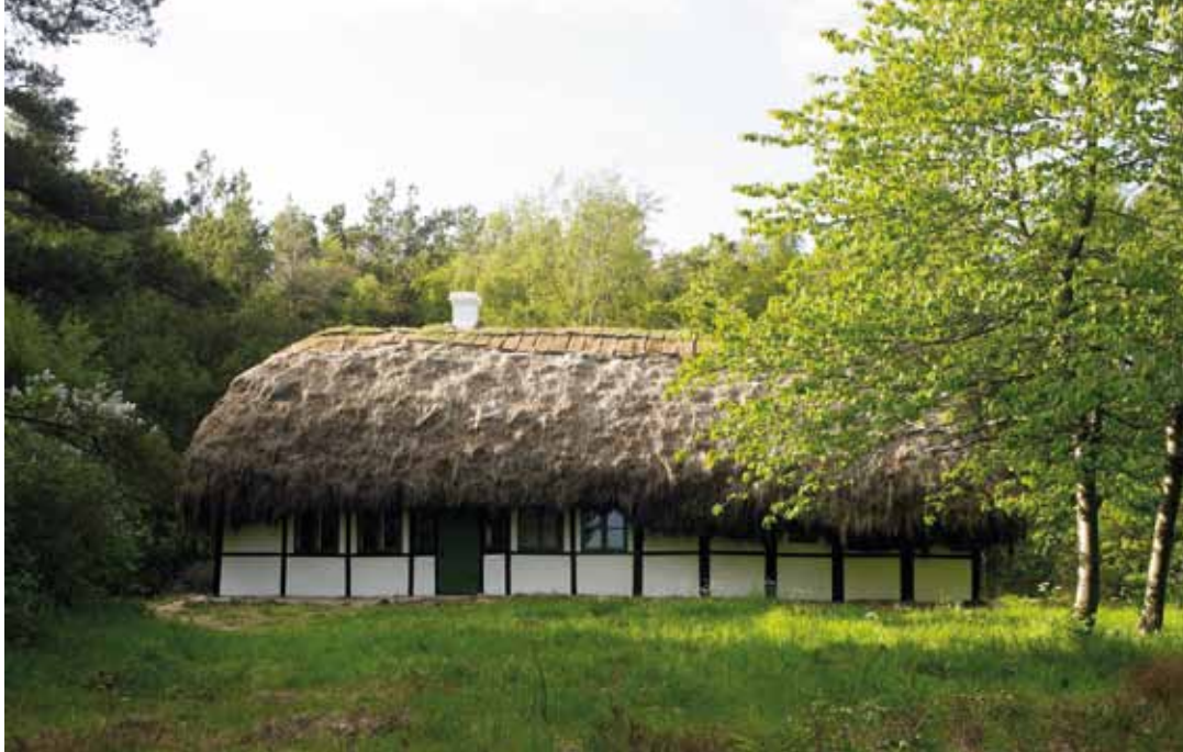
Kaline's House – an old seaweed-thatched house placed on Læsø, a small island in the northern Kattegat.
