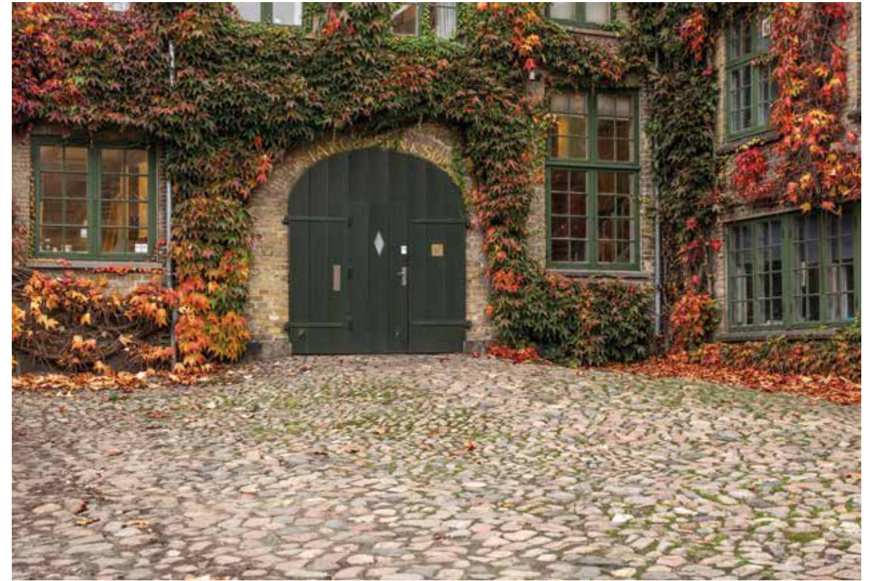
Marcussen's House – a historic industrial site with buildings dating from three centuries.
